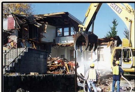
Demolition of homes taken by Eminent Domain in New London.
